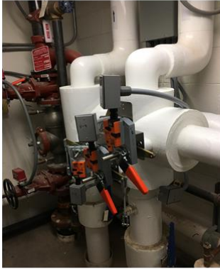
Installation of bypass valves
