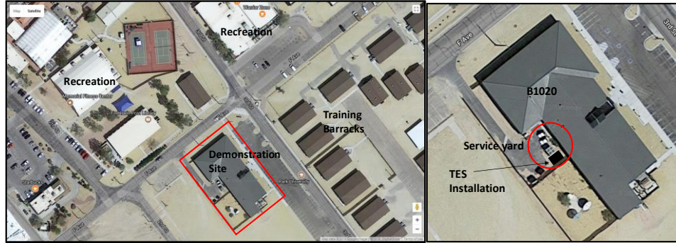
Figure 12. Aerial images of building street location and TES installation in rear service yard
