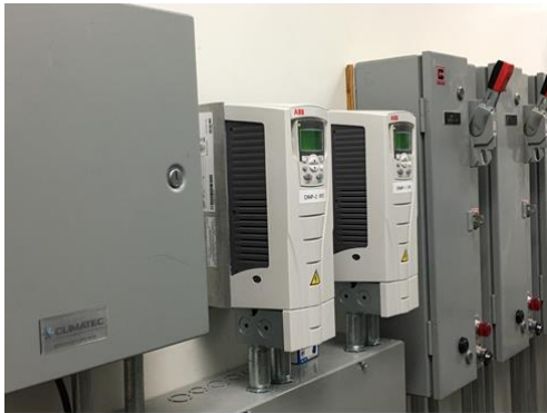
Installation of VFD's to CHW pumps
