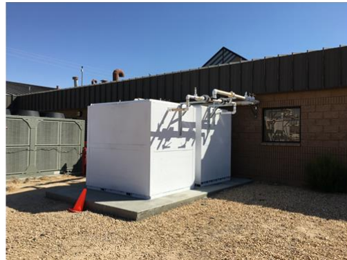
Figure 14. INSTALLATION IMAGES for Phase 1
