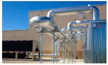
PhaseStor thermal storage system can help with short cycling for chillers, boilers and shift peak demand load when electrical rates are at a premium.
