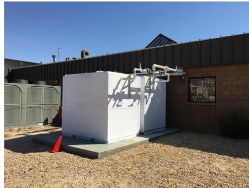
Figure 14. INSTALLATION IMAGES for Phase 1
