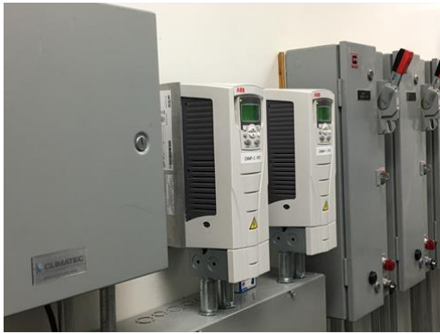
Installation of VFD's to CHW pumps
