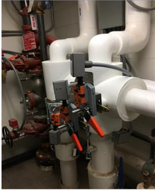
Installation of bypass valves
